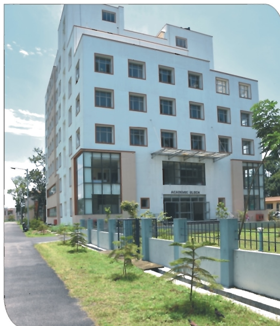
Photo: Infrastructure Development Work
